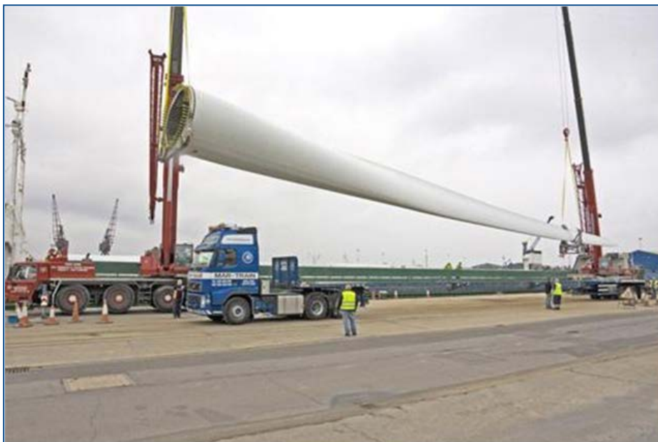
Figure 16.4: Unloading of Wind Turbine Blade
