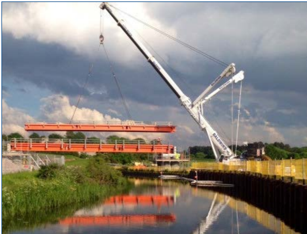
Figure 16.7: Temporary Bridge – Typical Installation
