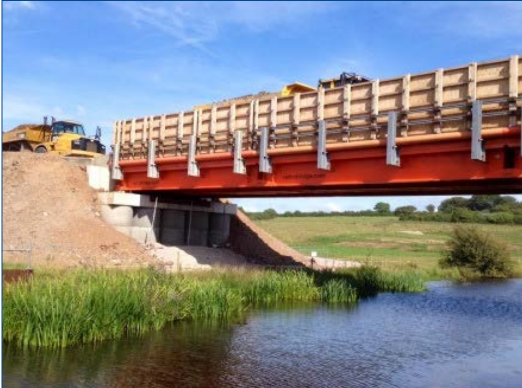
Figure 16.6: Temporary Bridge – Typical View
